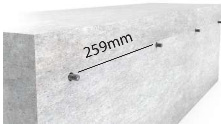
1. Drill, vacuum, insert glue and chemical anchor.
